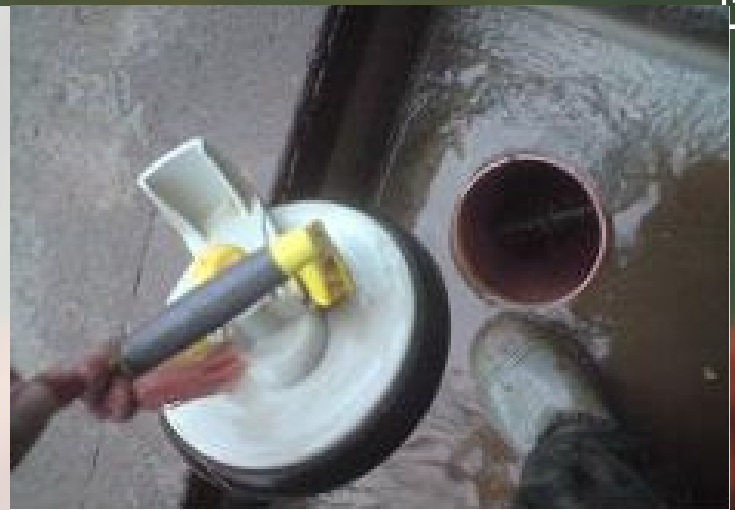
Fig 6: A 6" drain, bung and string pull
